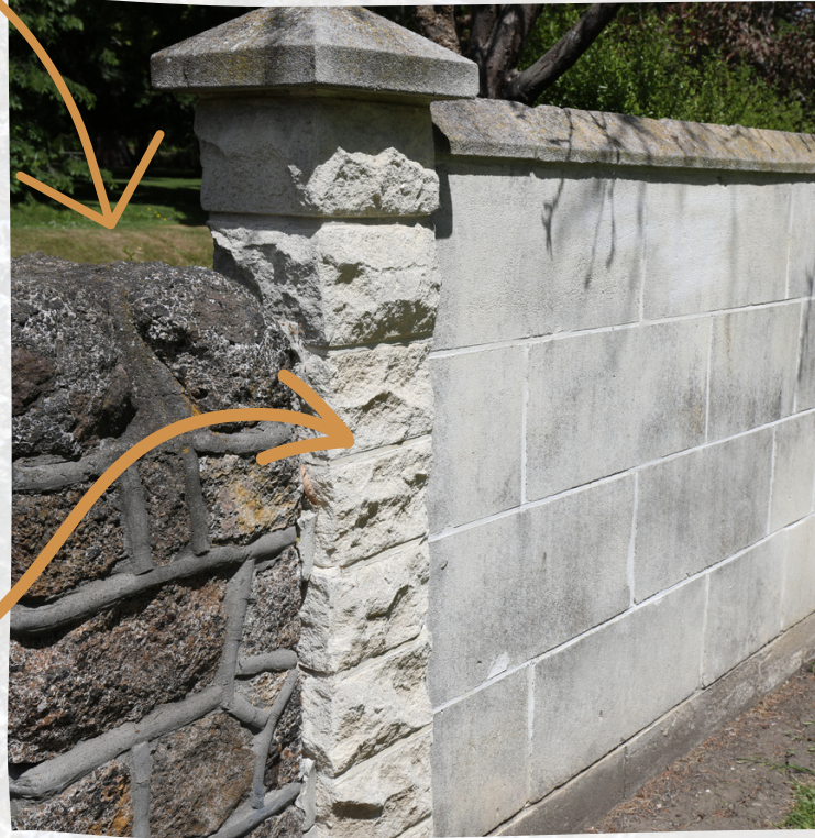
Wall at the Oamaru Public Gardens
